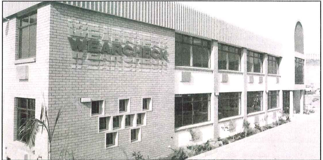
Impressive facade of Wearcheck's new head office and laboratory at Westmead, Pinetown.
