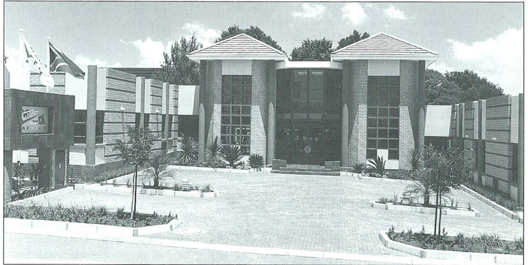
Wearcheck's new office building in Croydon, Johannesburg was completed at the end of last year.
