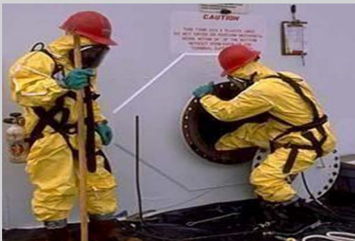
Technicians from Kenozi are seen here conducting cleaning of petroleum storage tanks
